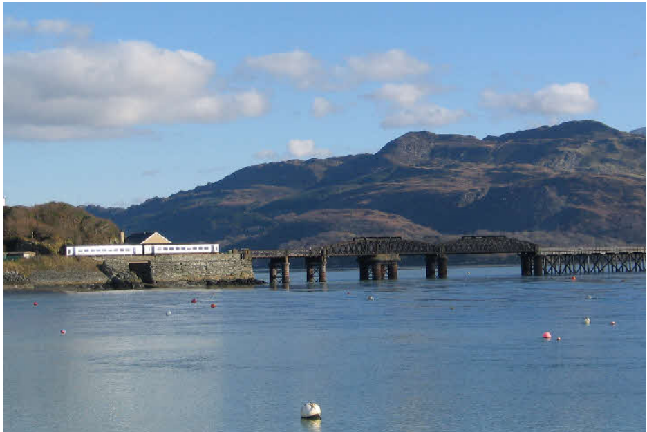
The Heart of the Coast Line. An up train crosses the Barmouth Viaduct on the 6th February 2007.
